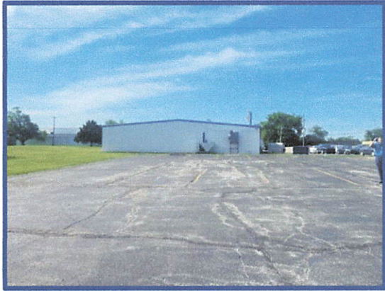
Exterior view of 300 North Marion Street (Building 2) facing south
