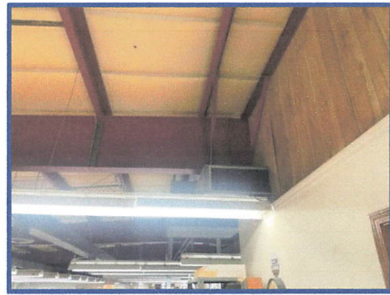
Interior view of Building 2's ceiling
