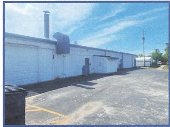
Exterior view of 300 North Marion Street facing southeast
