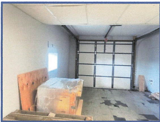
Interior view of storage area/dock door in Building 1
