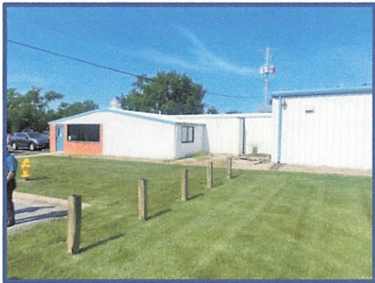
Exterior view of 249 North Troost (Building 3), 300 North Marion Street, & corridor facing southwest
