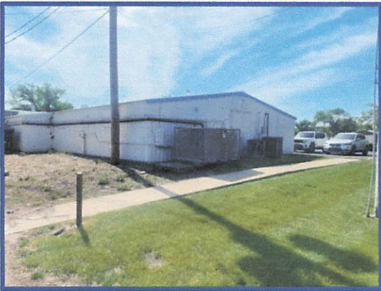
Exterior view of 249 North Troost Street facing southeast
