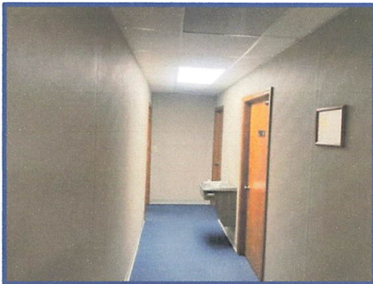
Interior view of bathroom entrance in Building 1
