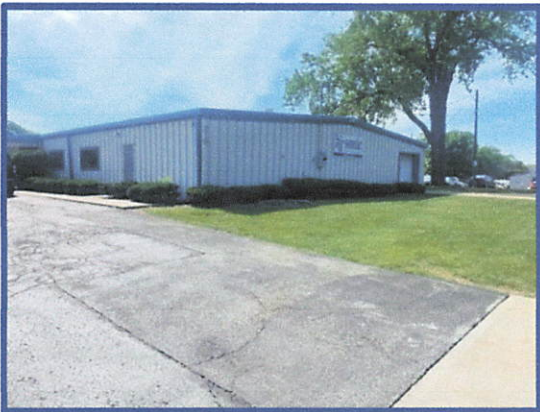
Exterior view of 310 North Marion Street (Building 1) facing east
