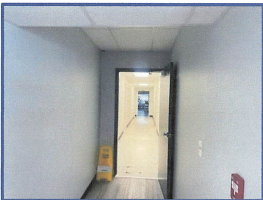
Interior view of connecting corridor from Building 3 facing north towards Building 2
